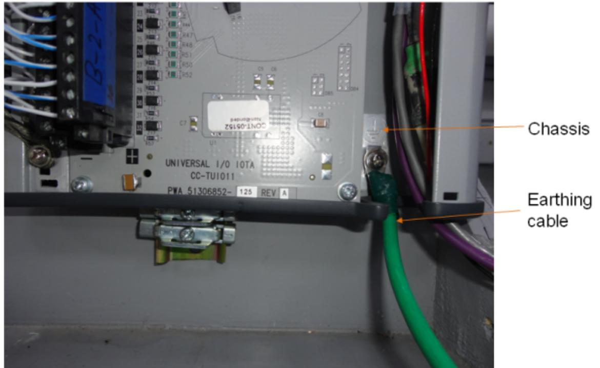
Figure 164: Grounding connections
