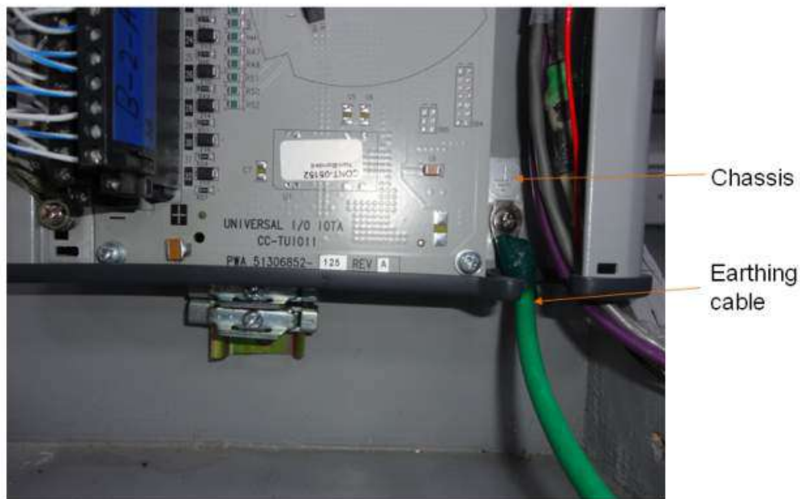
Figure 164: Grounding connections
